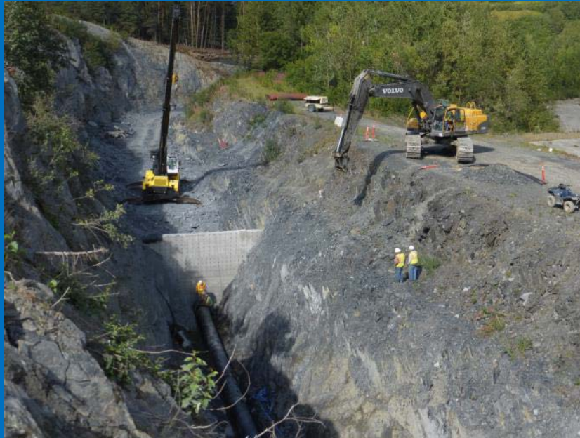
Siphon Pipe installation – August 2014
